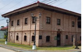
Restoration works done at the main house covered the rehabilitation of existing clay roof tiles and general repainting. At the E-Learning building, maintenance works included the replacement of damaged roof tiles and waterproofing works, ceiling works, electrical works, replacement and repair of the existing well and trench drain basin, and repainting of the existing perimeter fence.
